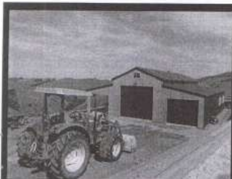
Recently constructed 14 x 16 x 4.2m American Barn with ply & batten cladding on end wall and internal dividing wall. Built near Matamata, this shed utilises a partial clear span design to provide an unobstructed work shop area.
