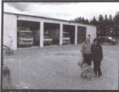
Adjusting the bay widths on this shed used by a food distribution business reduced waste space between the trucks and increased valuable storage space.
